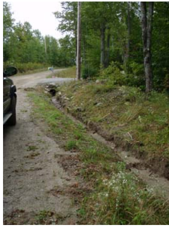
Cove Way Site 7 Before
