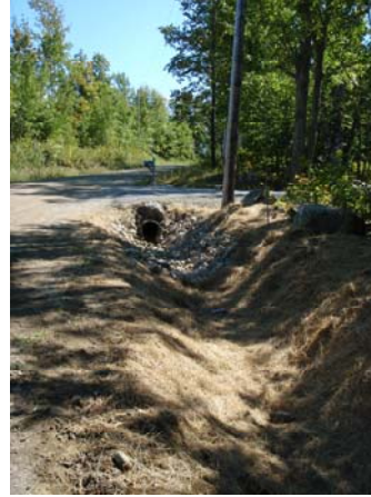
Cove Way Site 7 After
