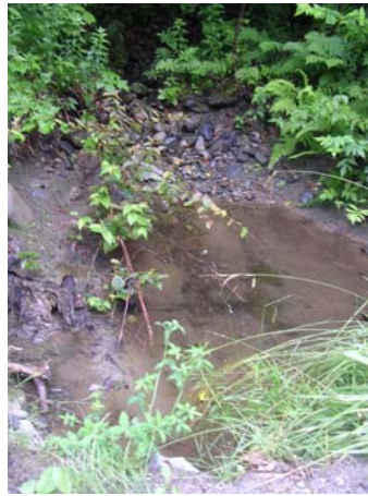
Cove Way Site 3 Before
