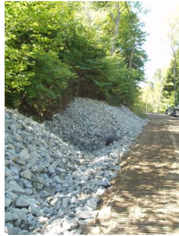
Cove Way Site 3 After
