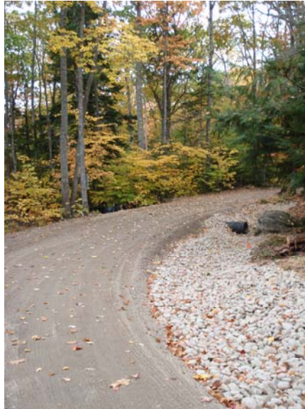
Walls Farm Way After
