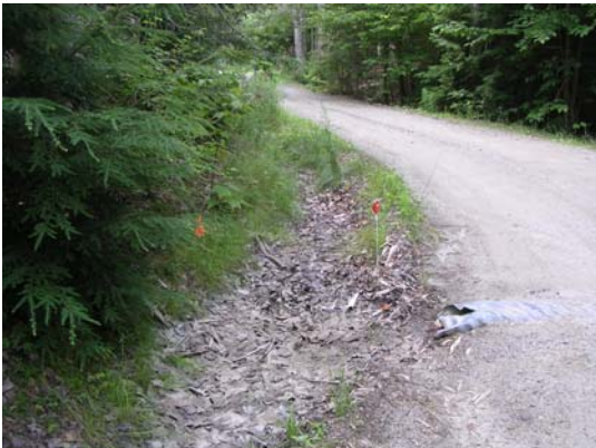
Wilson Way Site 2 Before
