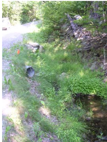
Phillips Way Site 2 Before
