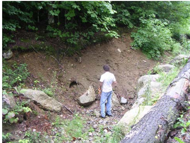
Cove Way Site 4 Before
