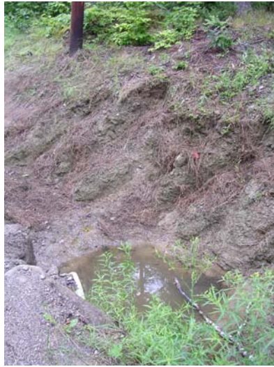
Cove Way Site 5 Before
