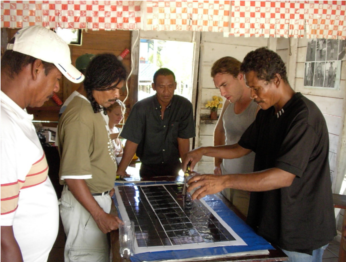
Photo 2 shows the group putting measured teaspoons of the expensive silicone on the PV cells. It will flow behind the cells and completely encapsulate them by capillary action.
