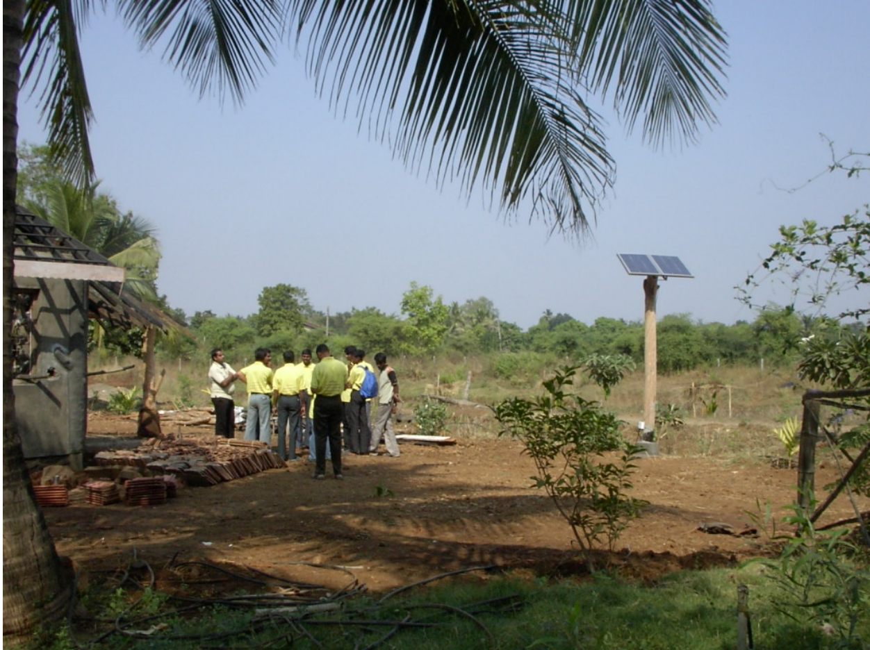
Photo 7, Installing the 120 watt PV system at the ecotourist resort.
